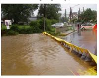
Water-inflated property protector (WIPP): Long tube barrier filled with water (very sturdy) ← protects homes from floods (effective as a barrier but does not dispose of the water)
