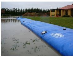
Flood barrier socks (Quick dam): Small, sandless sandbags (efficient and easy to use) ← very popular \*not practical for large floods
