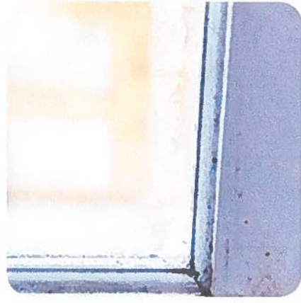
Peeling caulk or grout
