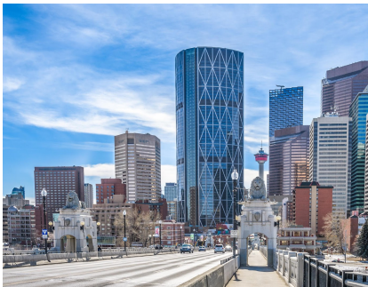
Stormwater management - Calgary
